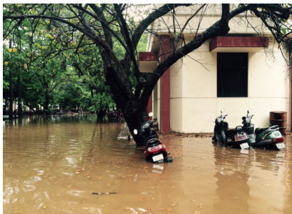
Inundation of IITM-campus after a flash flood in April 2015
